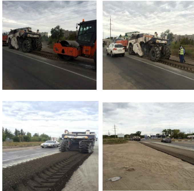
Fig.1 Implementation of operations on thin layer road structures by the method of cold regeneration. 2015
