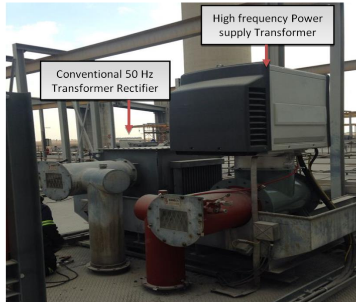
Figure 4: New HFPS transformer installation.
