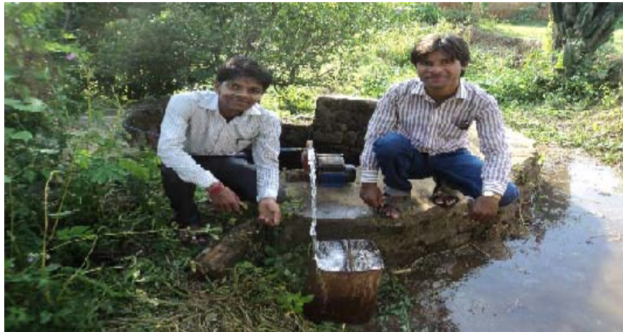
Fig. 4: The hybrid powered water pump to deliver water from the well.
