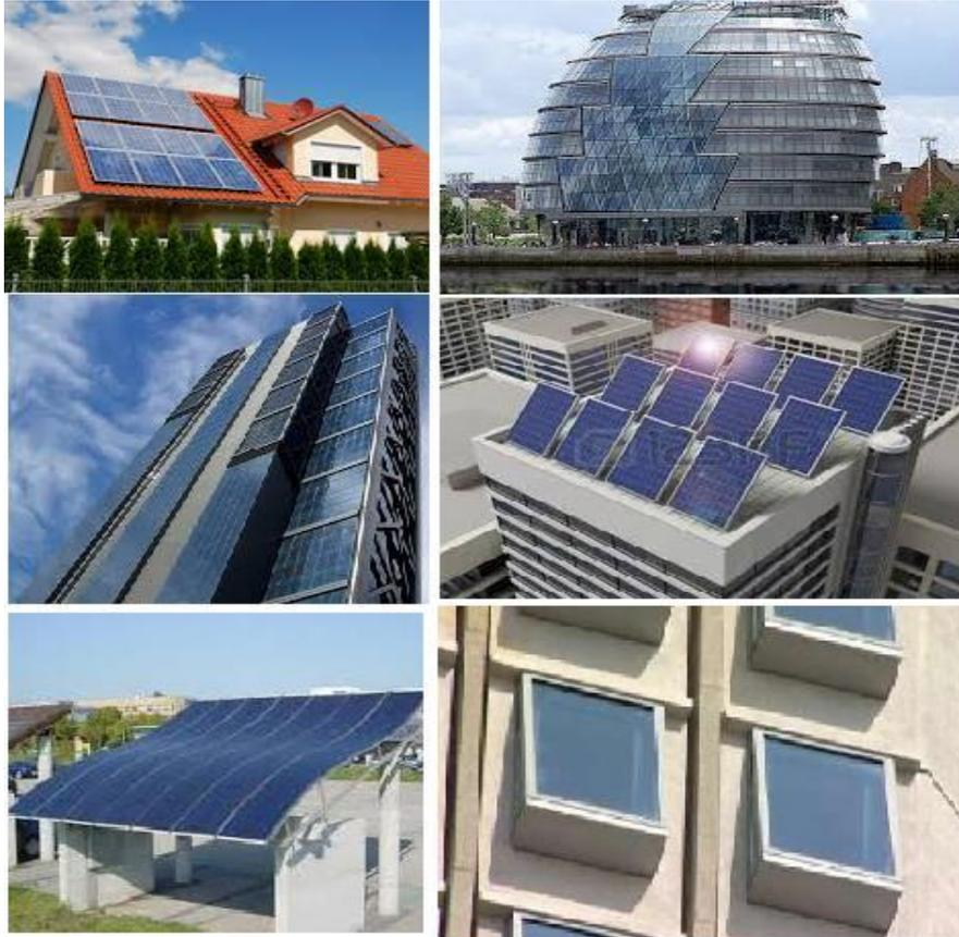
**Figure 7:** Different ways for installing the solar panels using the exterior building elements
