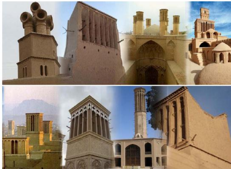
Figure 3 : Several ancient wind catchers with different configurations [4].
