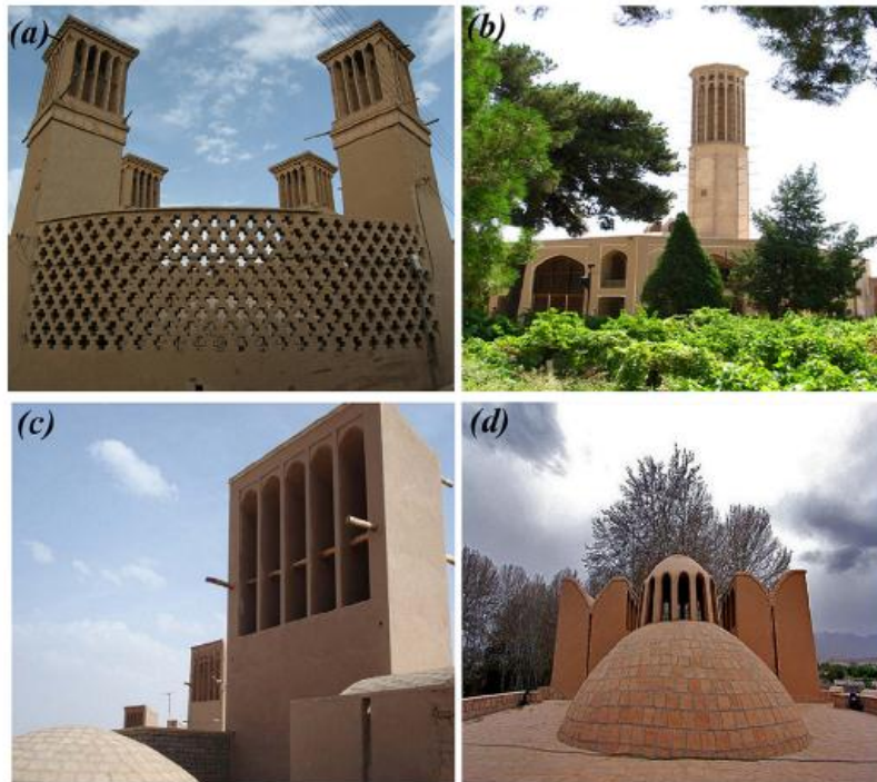
Figure 2 : Several wind-catchers with different configurations, (a) four-sided wind-catcher with flat roof (Yazd), (b) octahedral-sided wind-catcher with flat roof (Yazd), (c) one-sided wind catcher with steep roof (Ardakan), (d) two-sided wind catcher with curved roof (Mehriz) [3].
