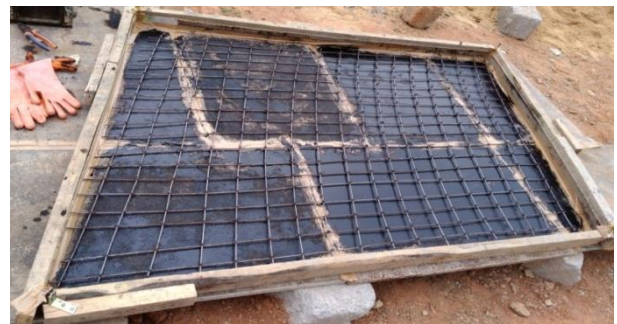
Figure 3: Typical Layout of Reinforcement Cage
