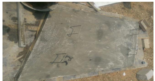
Figure 4: Casting of a Typical Skew Slab
