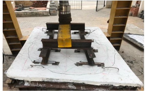
Figure 7: Typical Cracking Pattern of Skew Slabs on Compression Side
