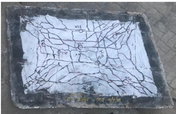
Figure 6: Typical Cracking Pattern of Skew Slabs on Tension Side
