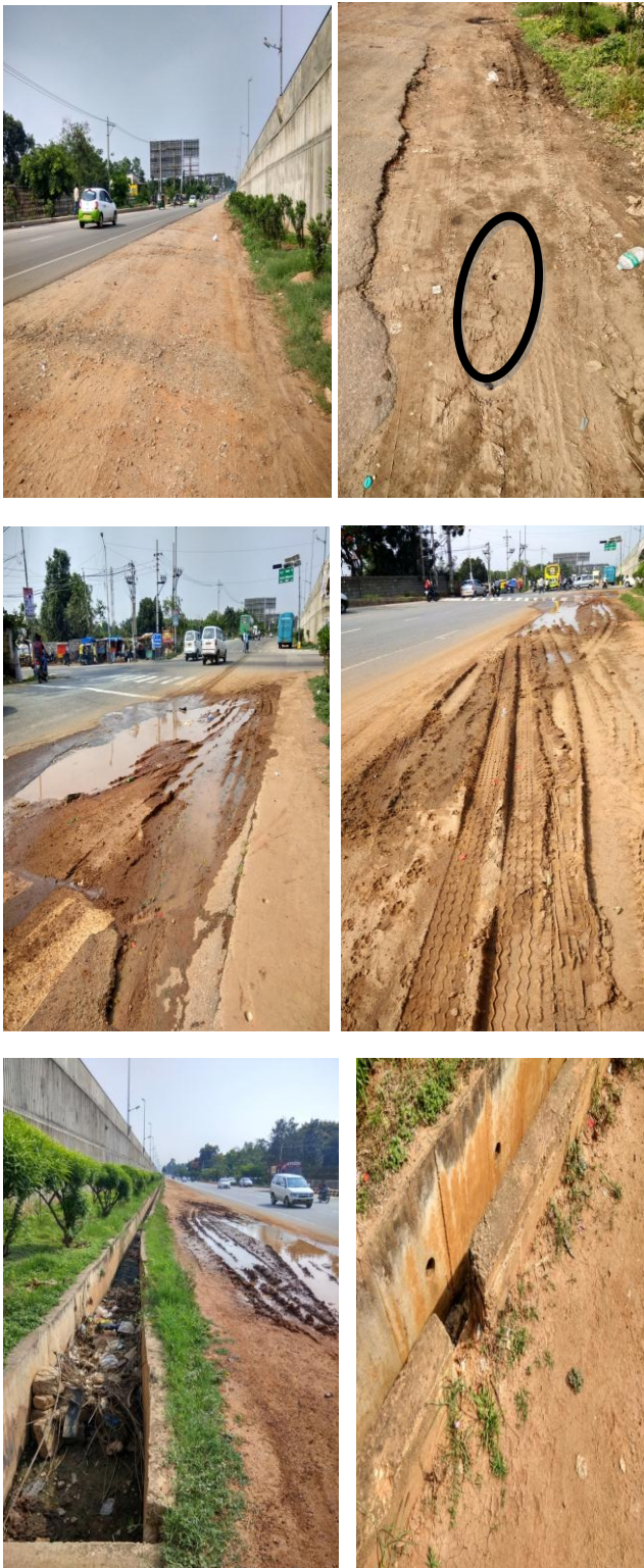
Fig-4: various shoulder failures and causes at Bagaluru Cross
