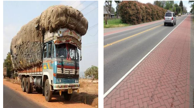
Fig-2: Unpaved and paved shoulder
