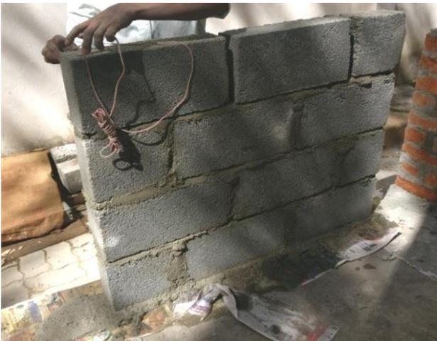
**Figure 2 :** Casting of Solid concrete block masonry wall
