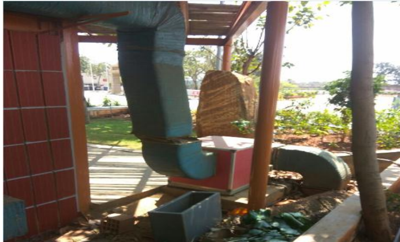
Figure 4: Passive cooling system
