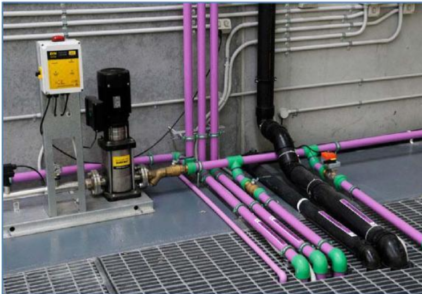
Figure 3: International examples of colour coding of pipes for recycled water
