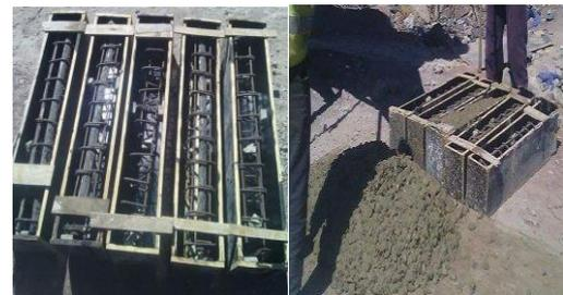
Figure 2. Fresh concrete mix and reinforcement
