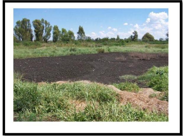
**Figure 3:** Example of maturation pond filled with sludge (Snyman et al.,2006)
