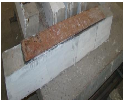
Figure 6. GFRP sandwich panel bonded to the soffit of the beam using polyester resin
