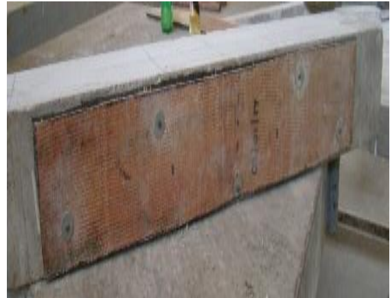
Figure 7. GFRP sandwich panel bolted to the soffit of the beam using screws & washers
