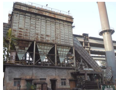
Figure 12. Picture of the 12 Chamber Filter Bag Unit
