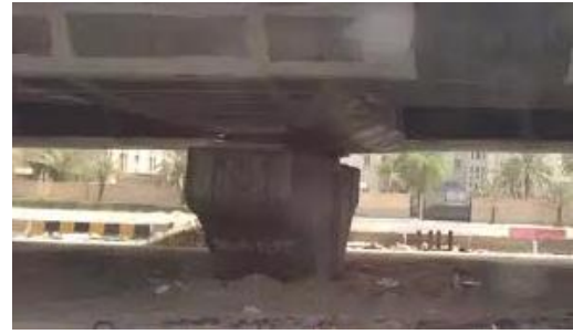
Figure 6. Pier: Lower (first layer) supporting superstructure
