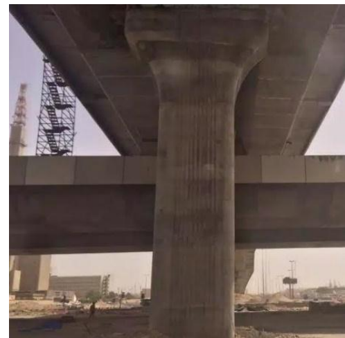
Figure 8. Pier: Second layer of superstructure
