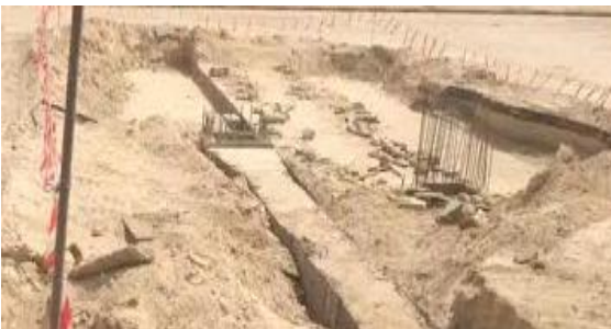
Figure 4. Superstructure where the upper bridge begin
