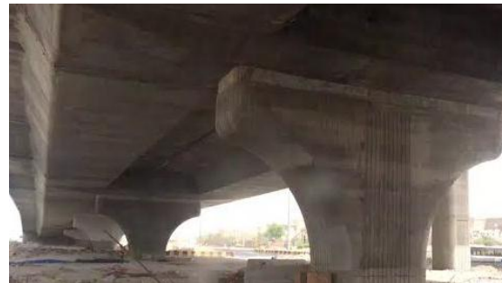
Figure 7. Pier: First layer of superstructure
