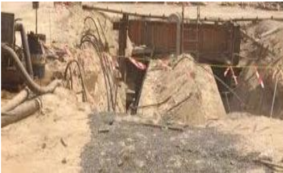
Figure 3. Initial processing of substructure
