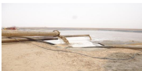
Figure 16: Waste pit (Drilling Y, 2017)
