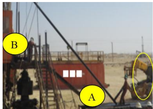
Figure 5: Conventional Catwalk, (Company X, 2017)
