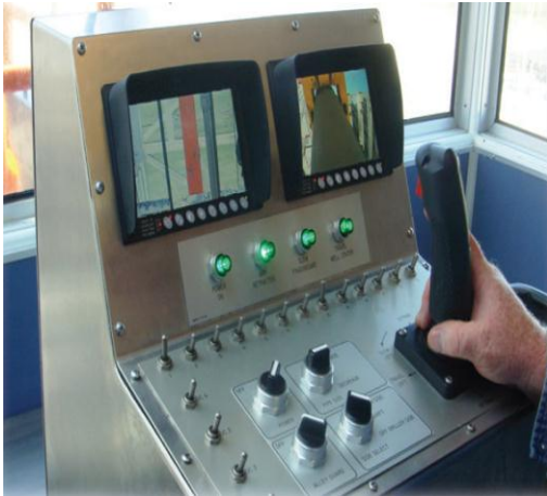
Figure 11: Iron derrick man operating panel (Keuri, 2017)
