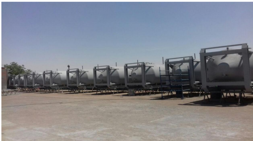
Figure 1: Silos after fabrication and painting
