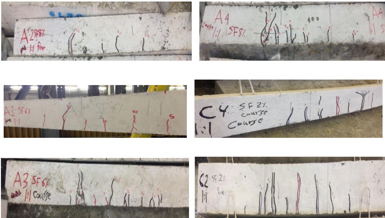
Figure 13 : Cracking of failure specimens for group 1 (C2,C4,A1,A2,A3,A4)
