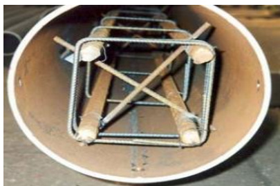
Figure 2: Concrete filled hollow section
