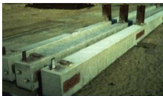
Figure 1: Concrete encased section
