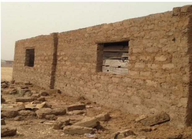
**Figure 4:** A recent construction using earth block walls
