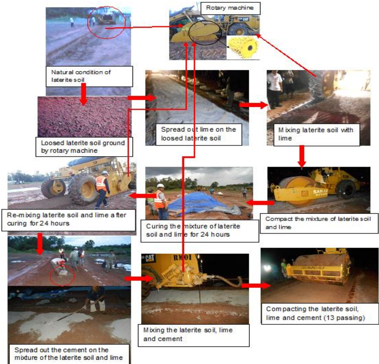
Figure 2. Mixing and compaction process on the field
