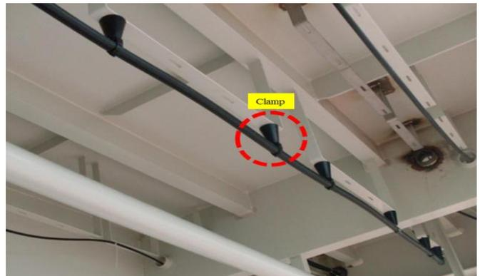
**Figure 8:** Installation of Leaky antenna
