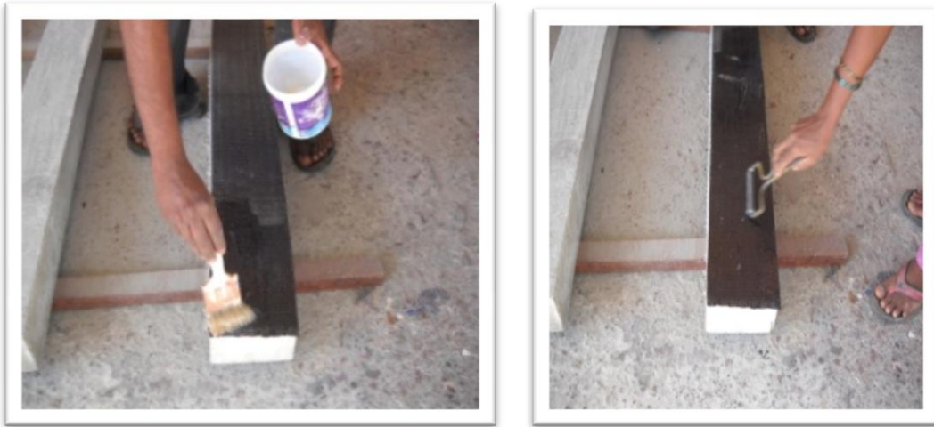
Figure 4: CFRP on the bottom of the beam
