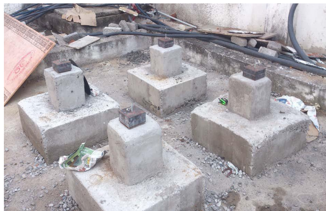
Figure 5: Fixing of elastomeric bearing with column
