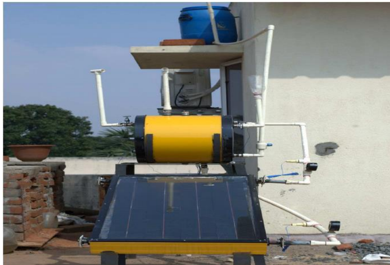
Fig.1. 25 LPD collector with primary riser tube and secondary storage tank
