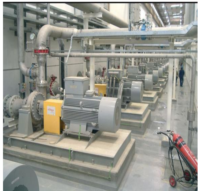
Fig.1. Motors used as pumps in the WTP
