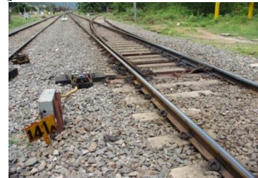
Figure 2. Point with DC motor
