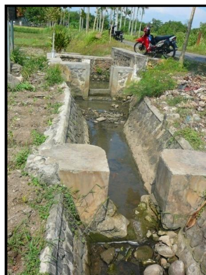
Figure 1: Broad Crested Weir in Tertiary channel with the Rupture Threshold
