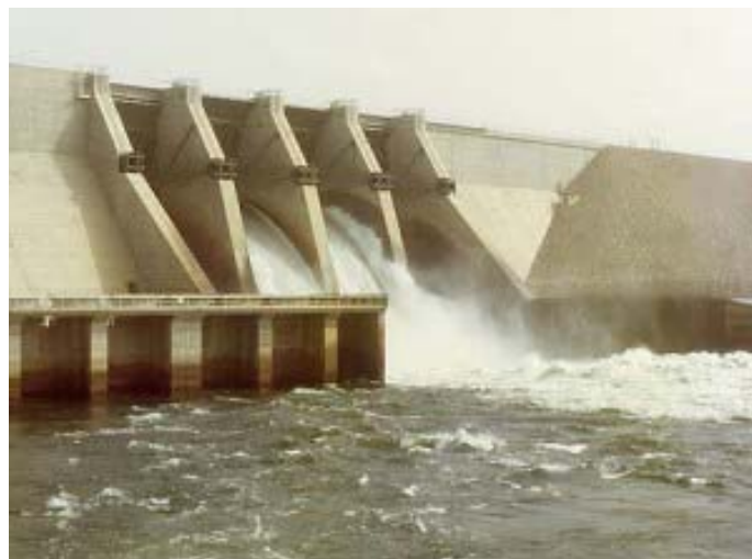
Fig. 1: Kainji dam located on River Niger, Northern Nigeria.
